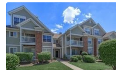
Legacy at Fox Valley Residential Location: Chicago, Illinois Apartment Units: 272
